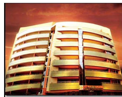
City Tower Bur Dubai
